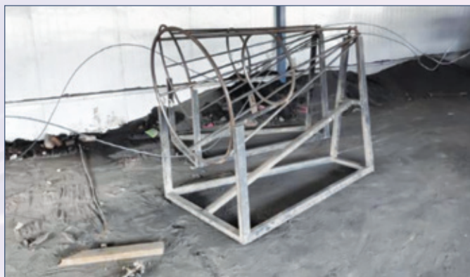
Protection for rebar straightening
