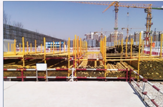
Material stacking rack
