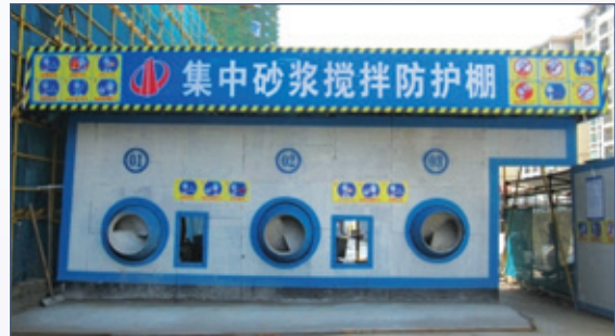
Setting up rain-proof and anti-smashing shed
