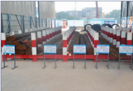
Rebar stacking rack
