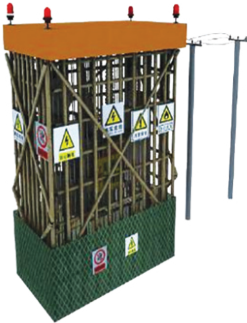
Protection for transformer
