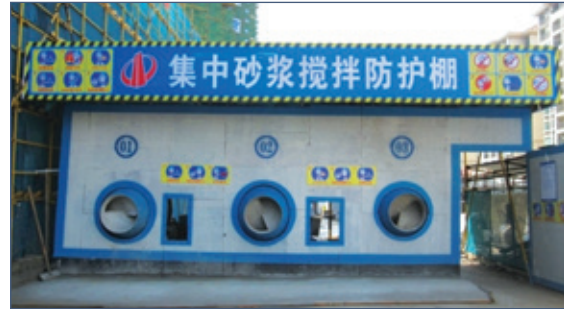
Setting up rain-proof and anti-smashing sheds
