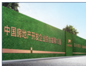
Fences at main exits and entrances
