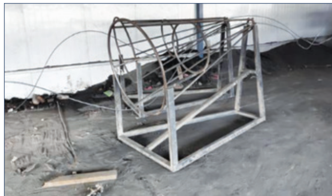
Protection for rebar straightening
