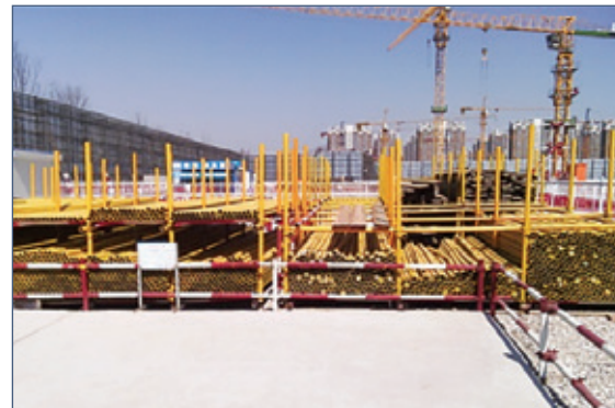
Material stacking rack
