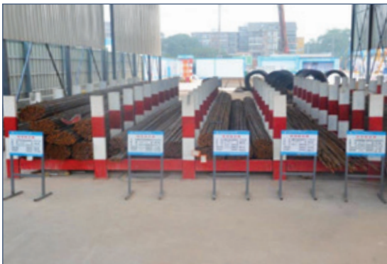
Rebar stacking rack
